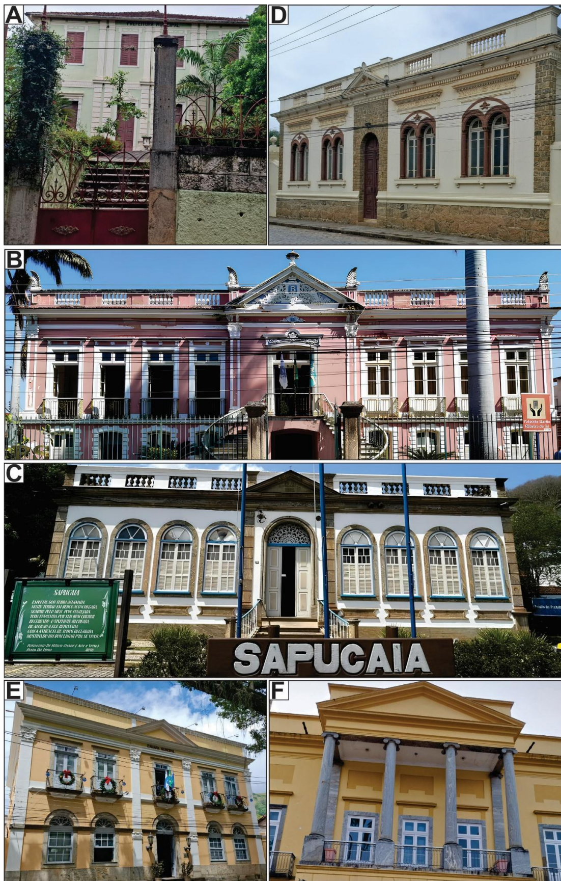
Fig. 11 Elite Residential Civic and Institucional Buildings: A. Além Paraíba Municipal Palace (MG); B. Barão Ribeiro de Sá Mansion, Paraiba do Sul (RJ); C. Sapucaia City Hall (RJ); D. Léa Pentagna House, Valença (RJ); E. City Council Valença (RJ); F. City Council Vassouras (RJ)
